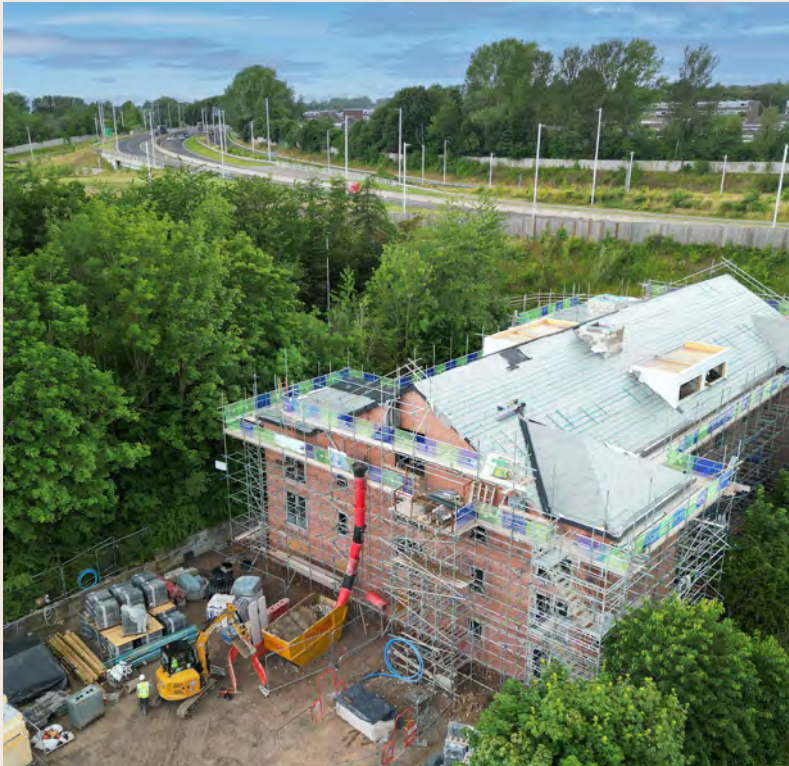
Front View of Hallwood Park, Eagles Way
