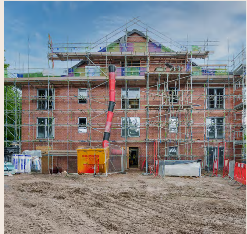
Front View of Hallwood Park, Eagles Way
