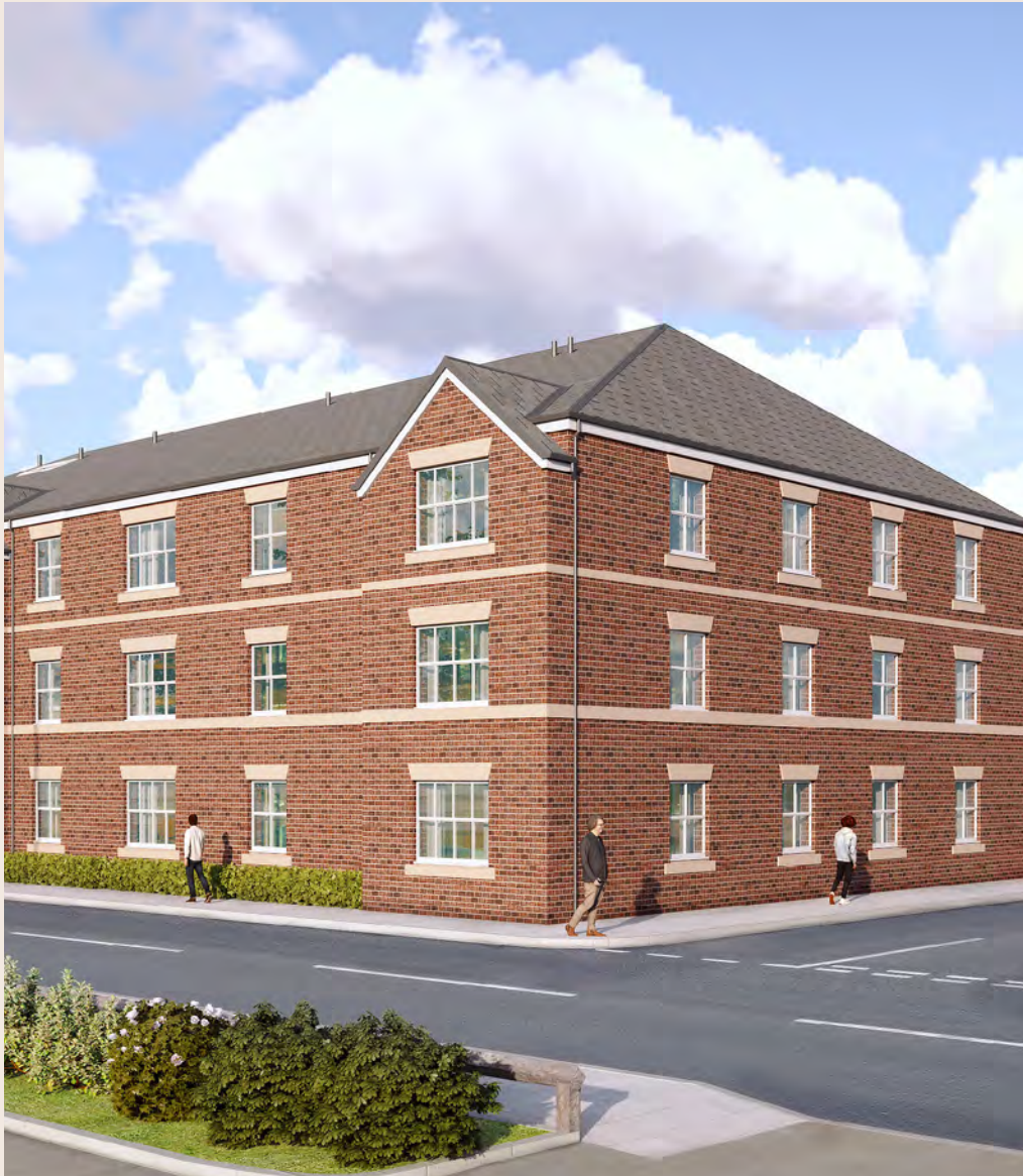
Marsh House, Manchester Road View
