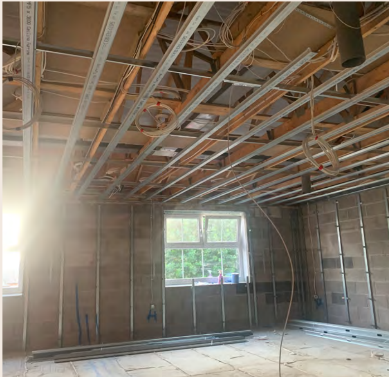
Internal Room Progression
