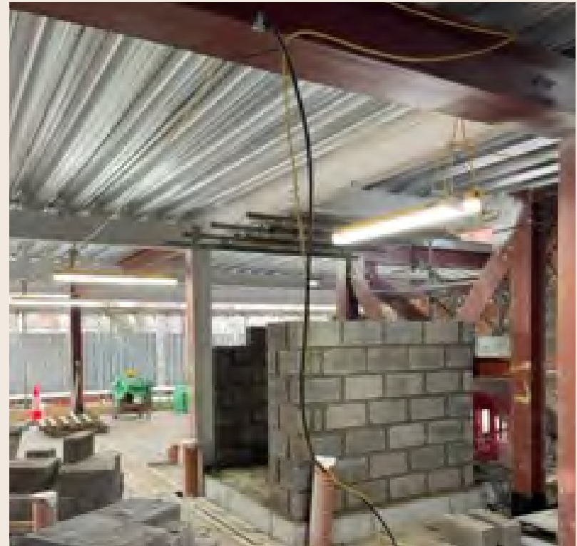
Lift Brickwork
