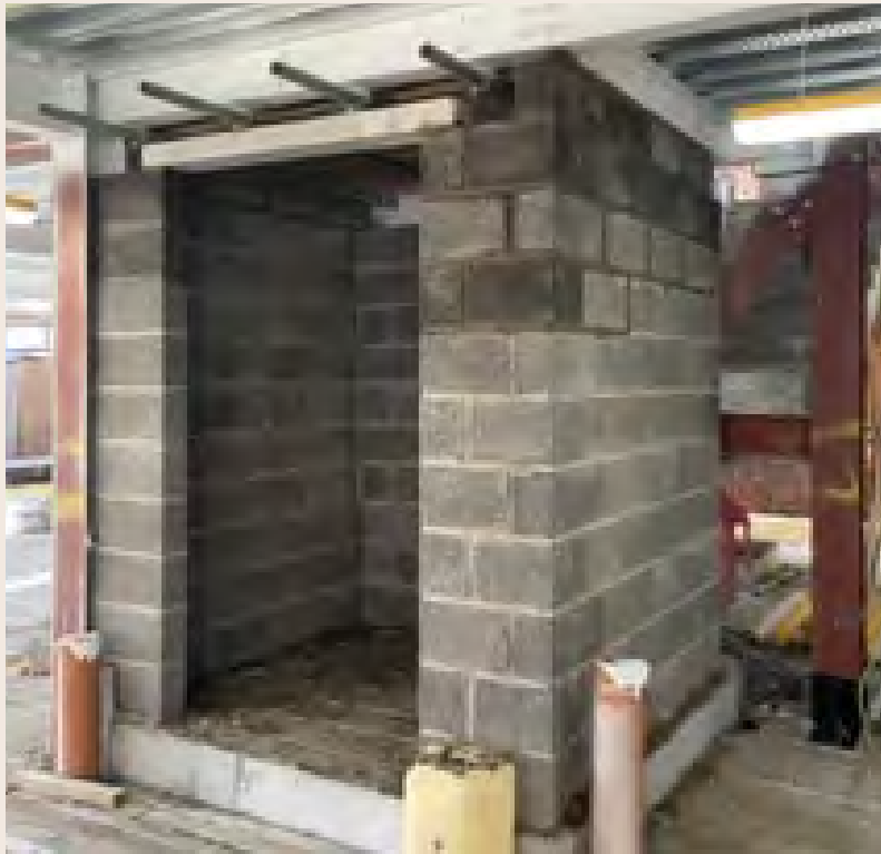
Lift Brickwork
