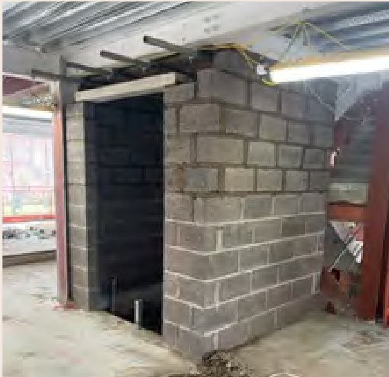
Lift Brickwork
