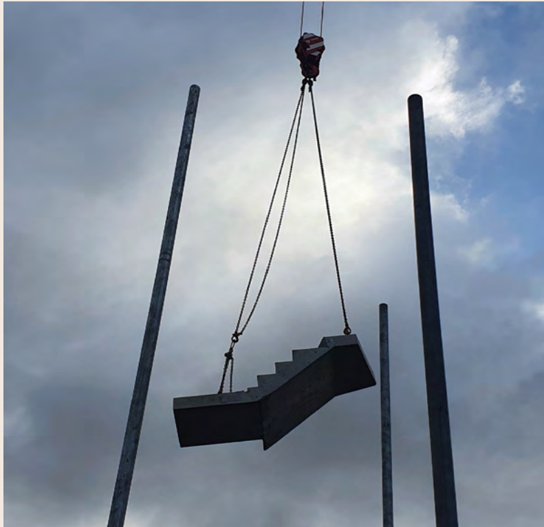
Stairwell Installation
